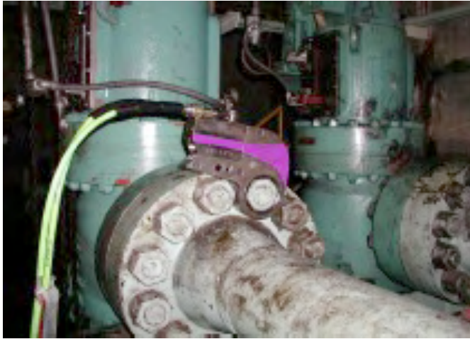
Finish Mill- Descaler Spray Valve Flanges Stealth-8 w 80mm link Torque 6700 Ft Lbs Torqued Pattern - 100%
