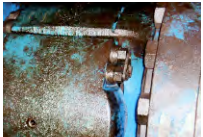
Hot Mill-Roll Shop- Cross Bearing bolts 8x1ct w (AB)60mm Link/Slider Torque- 6700 Ft. Lbs
